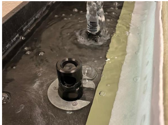
Figure 4. Specially made drain stopper (black cylinder) prevents over filling of the basin.
