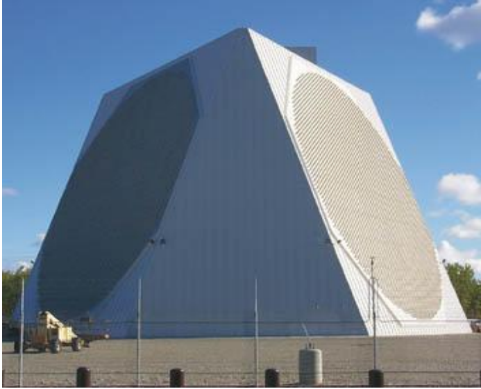
Fig. 1. A Giant Phased Array Radar in Alaska ( Courtesy of Alaska District, this 90-foot (27m) diameter radar installation monitors the northern sky. Its construction was part of the Clear Radar Upgrade to make all Ballistic Missile Early Warning System radars phased-array rather than mechanical. )
