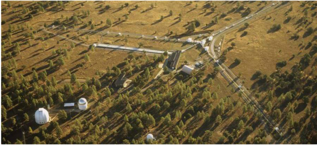
Fig. 1 Aerial view of the Navy Precision Optical Interferometer (NPOI) site, Flagstaff, Arizona (Photo courtesy of Michael Collier).
